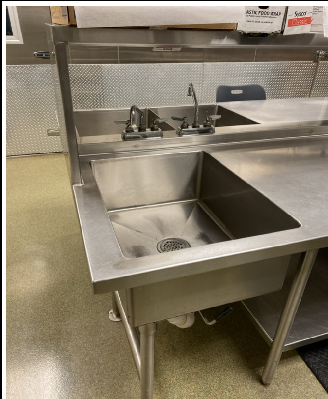
2/7/2024 - 1204-13 - Intermediate School - Kitchen - Southwest Sink
