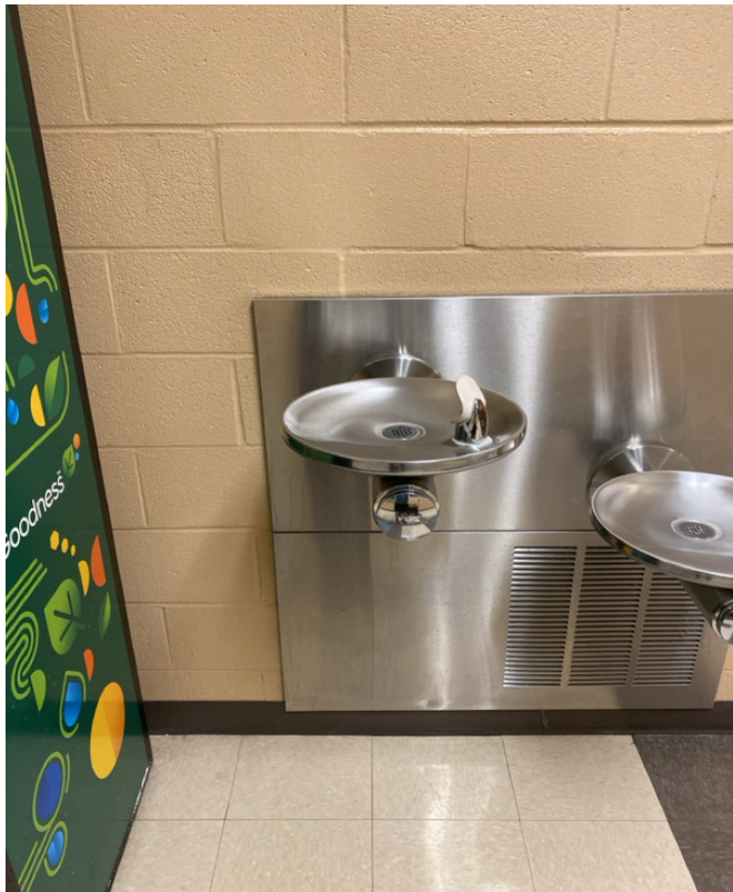
2/7/2024 - 1204-7 - Intermediate School - Outside Boys Restroom - Left
