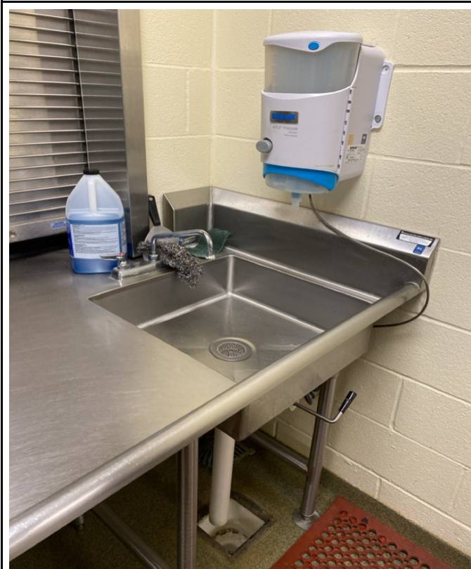
2/7/2024 - 1204-19 - Intermediate School - Kitchen - East Wall - Right
