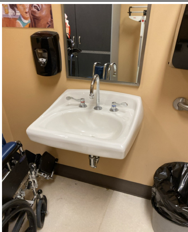
2/7/2024 - 1204-2 - Intermediate School - Nurse's Office - Restroom
